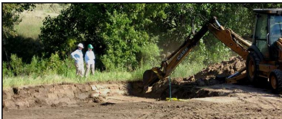
Figure 5-9. Crew Monitoring Stripping Process at 41PT245.
